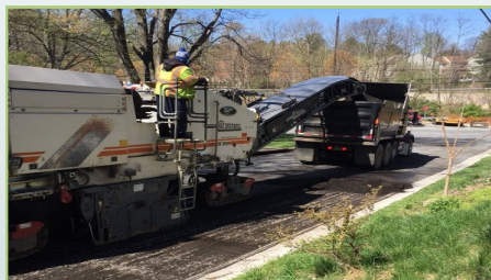
Milling machine patch excavating
