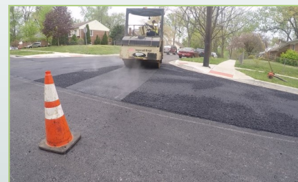
New asphalt is placed and compacted
