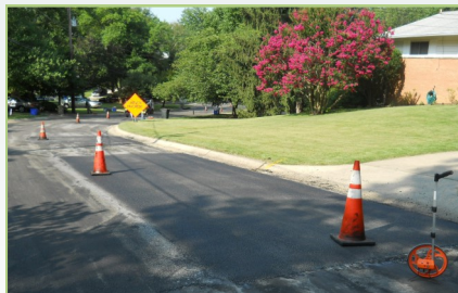
New patch is flush with existing pavement
